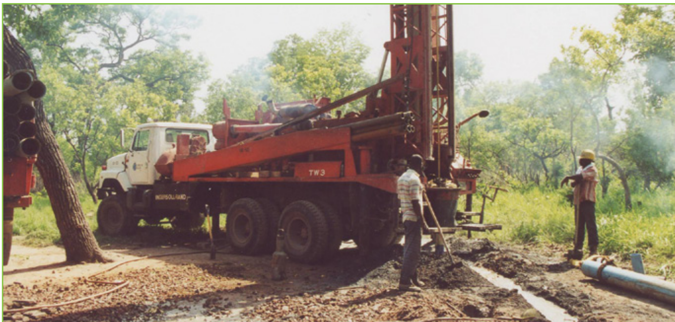
PICTURE ABOVE: Drilling a water supply borehole in Ghana
